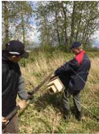
Ready to install Photo: Kirk Miles
