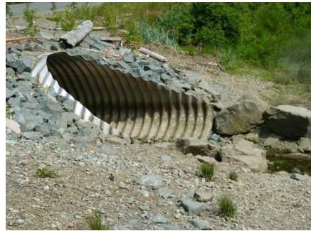
The installed culvert Photo: Kathy Masse
