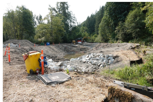
Fish pond excavators
